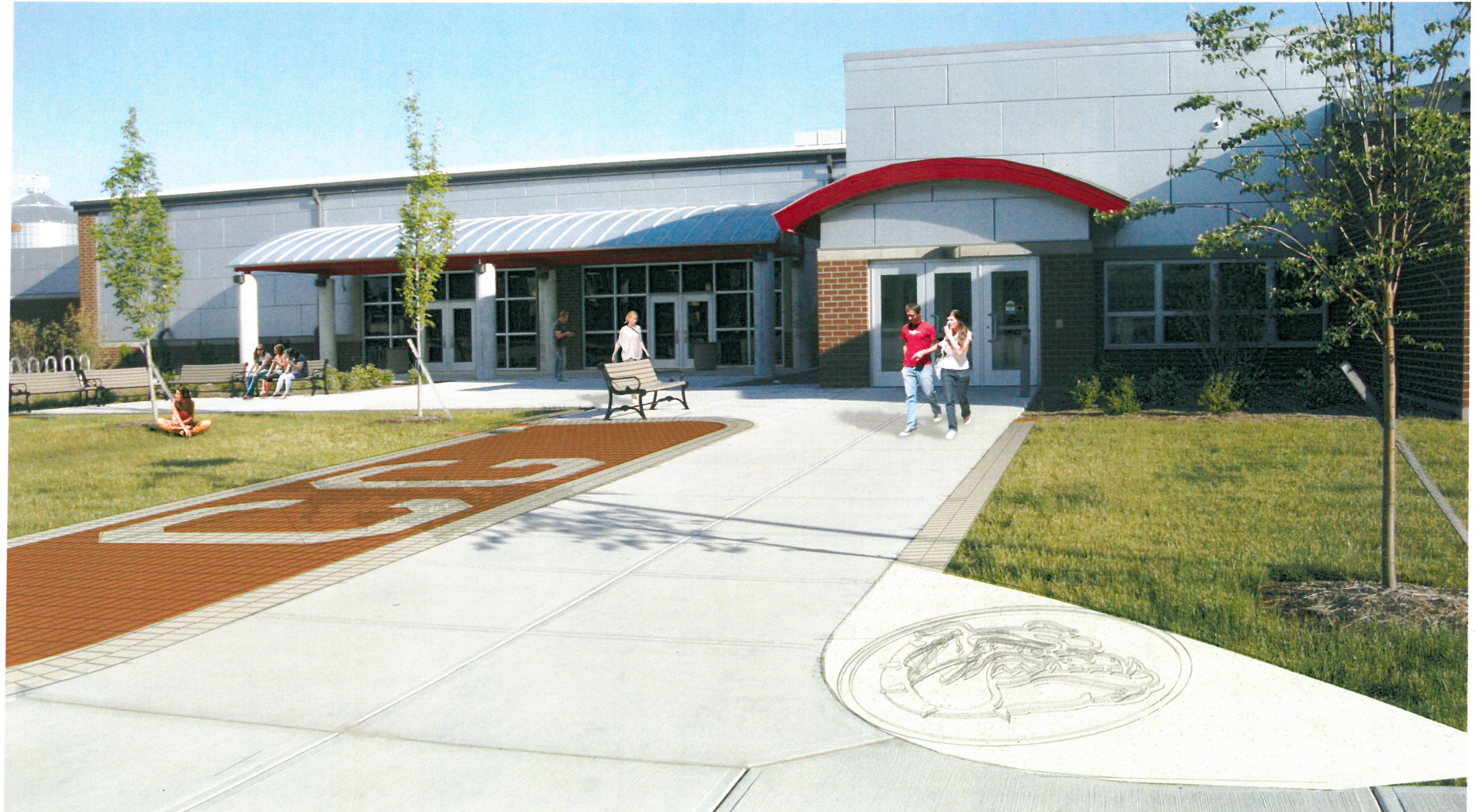
Columbus Grove High School Paver Patio Addition
